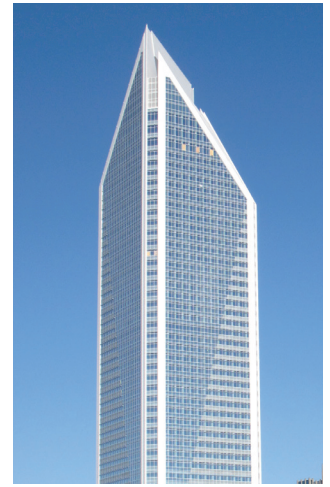
Featured Project: Duke Energy Center Charlotte, North Carolina.
